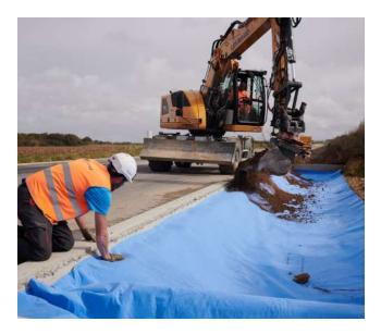
Designed for open-air and buried infiltration structures, **OSMORIA** Geoclean comes in three variants – Origin, Crystal, and Pure – allowing engineers to choose the appropriate level of filtration based on the expected pollution load.
