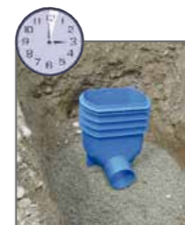
3. Min.: bedding in lean concrete mix
