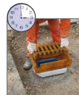
15. Min.: assembly of grating
