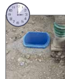
7. Min.: backfilling and compacting
