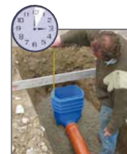
5. Min.: height adjustment
