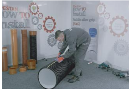
2. Determining position for montage
