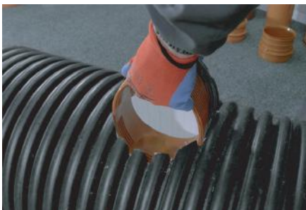
7. Inserting body of sag through pre-prepared opening and setting it in the appropriate position
