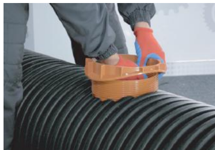
8. setting the spacer ring
