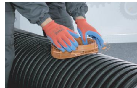
9. Tightening the sag
