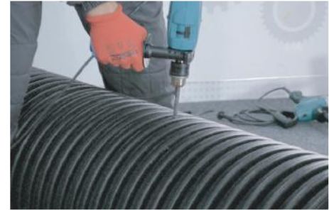
3. Drilling holes for the guided crown saw
