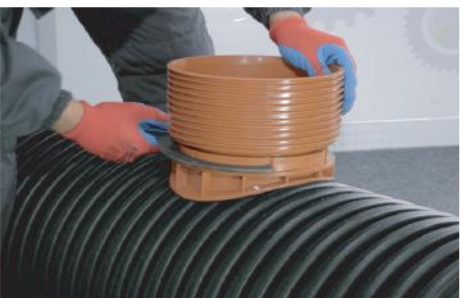
12. Final tightening of sag
