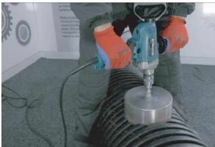
4. Drilling holes with crown saw
