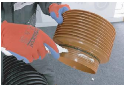
10. Lubricating appropriate connection of sag
