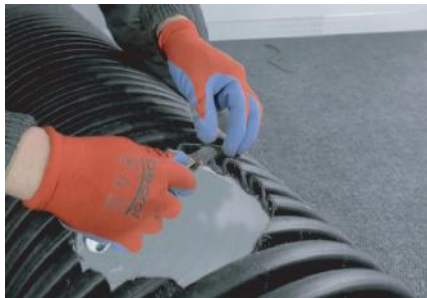
5. Cleaning chips and forming a clear hole
